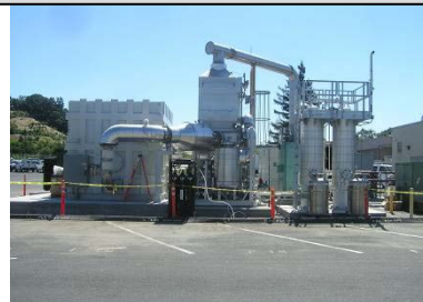
1.4 MW plant at a municipal building
