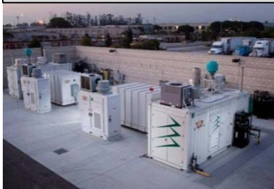
600 kW plant at a food processor
